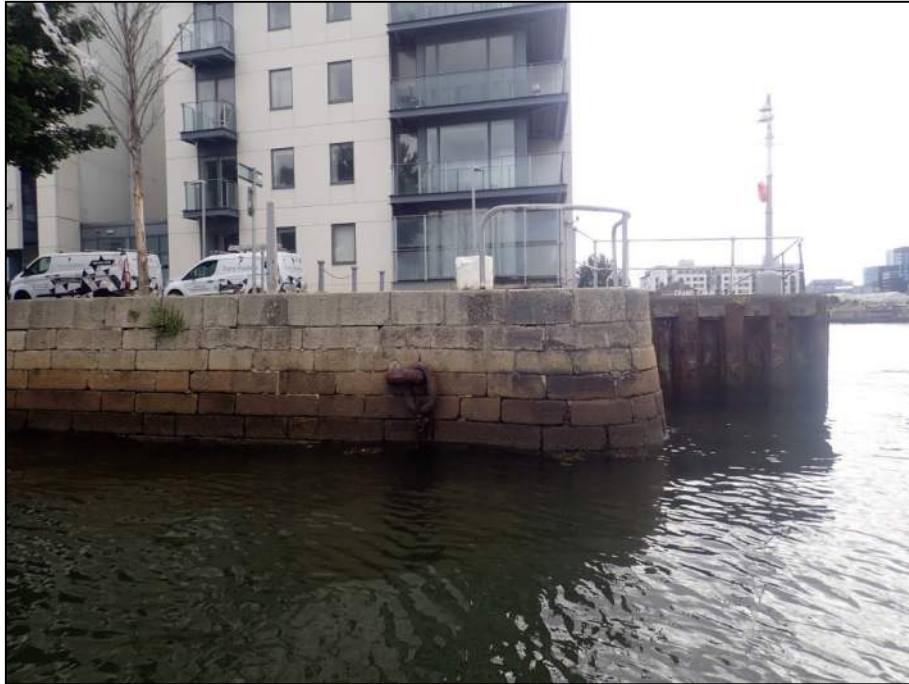
Plate 23: South-facing view of masonry quay wall and associated mooring ring, located at ITM 717924E, 734211N.
