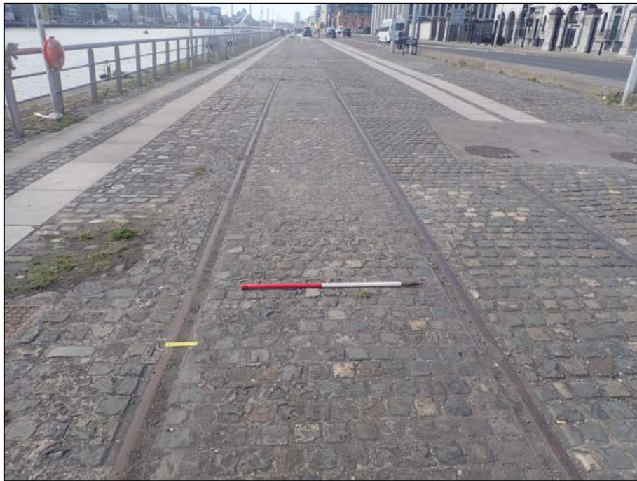
Plate 19: West-facing view along campshire at North Wall Quay, note iron-rails associated with goods carriages (1m scale).
