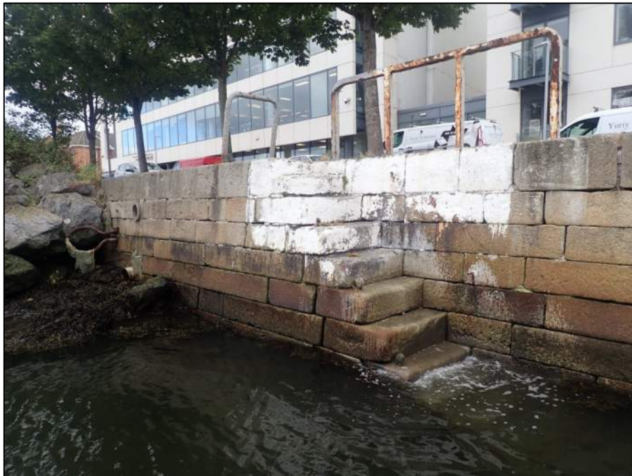
Plate 24: Southeast-facing view of a flight of river access steps located at ITM 717932E, 734208N.
