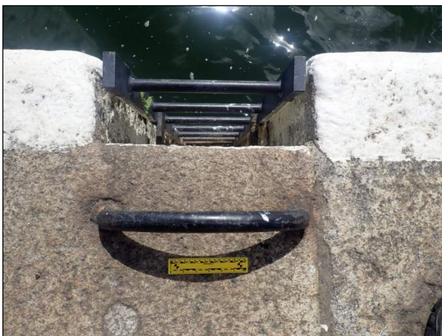
Plate 12: Recessed river access ladder (AL01), located at ITM 717965E, 734391N (150mm scale).
