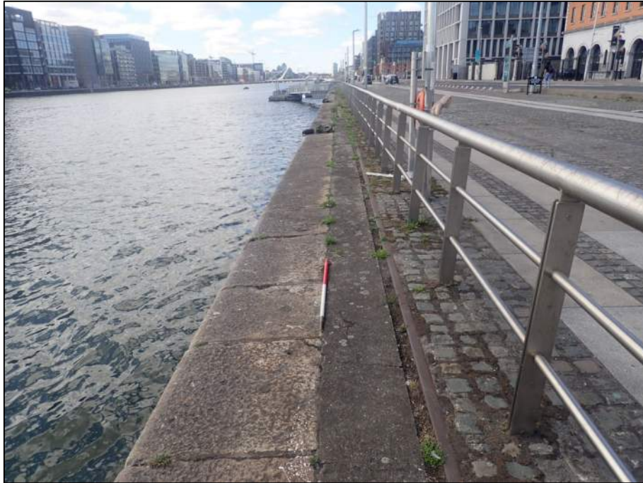
Plate 7: West-facing view along top of the North Wall Quay, showing large granite capping stones and section of crane-rail located behind (1m scale).
