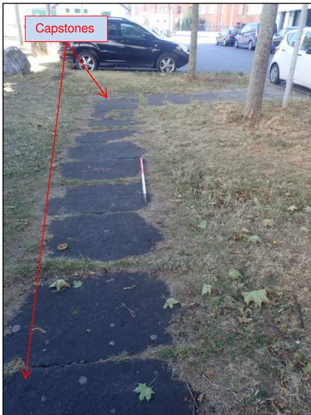
Plate 22: East-facing view at point where the unnamed quay becomes buried within area of reclamation (1m scale).
