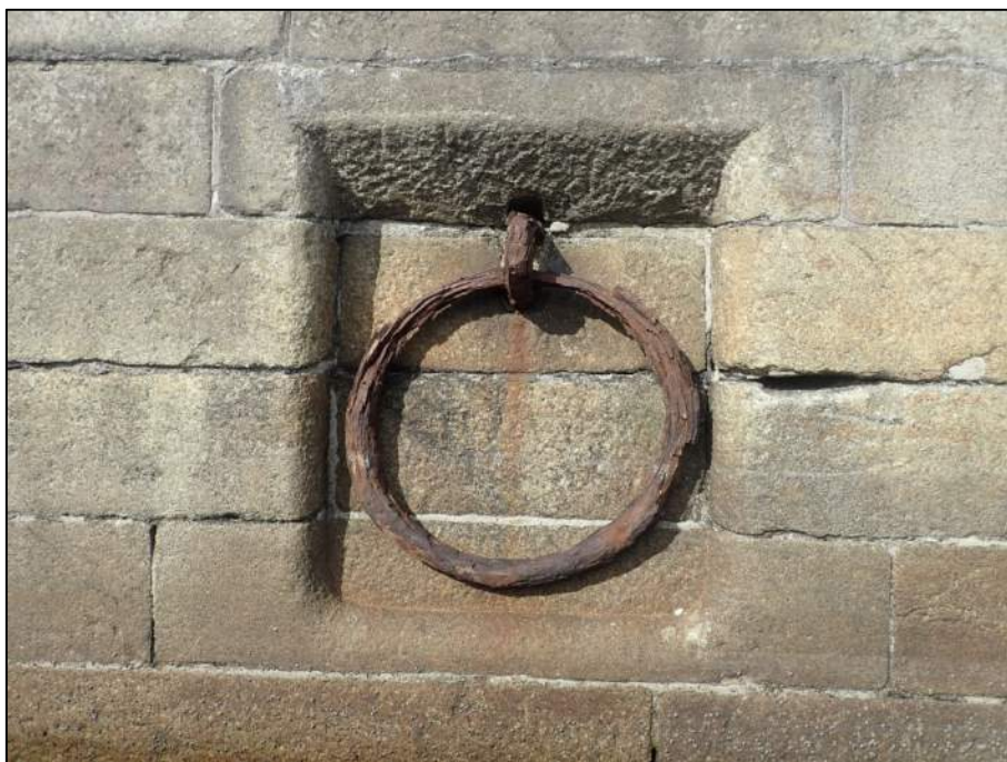
Plate 13: Recessed mooring ring (MR01), located at ITM 717990E, 734388N.
