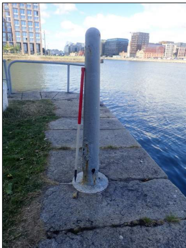
Plate 26: Partial remains of a derrick or similar lifting structure, inset into capstone area of quay wall (1m scale).
