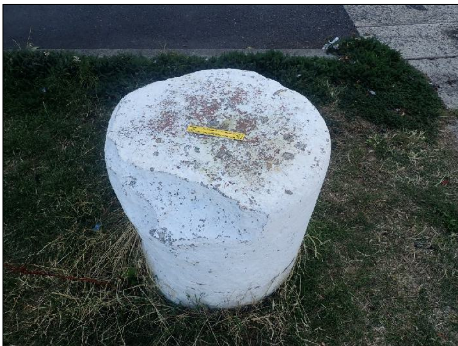
Plate 25: Mooring bollard located at ITM 717928E, 734209N (150mm scale).
