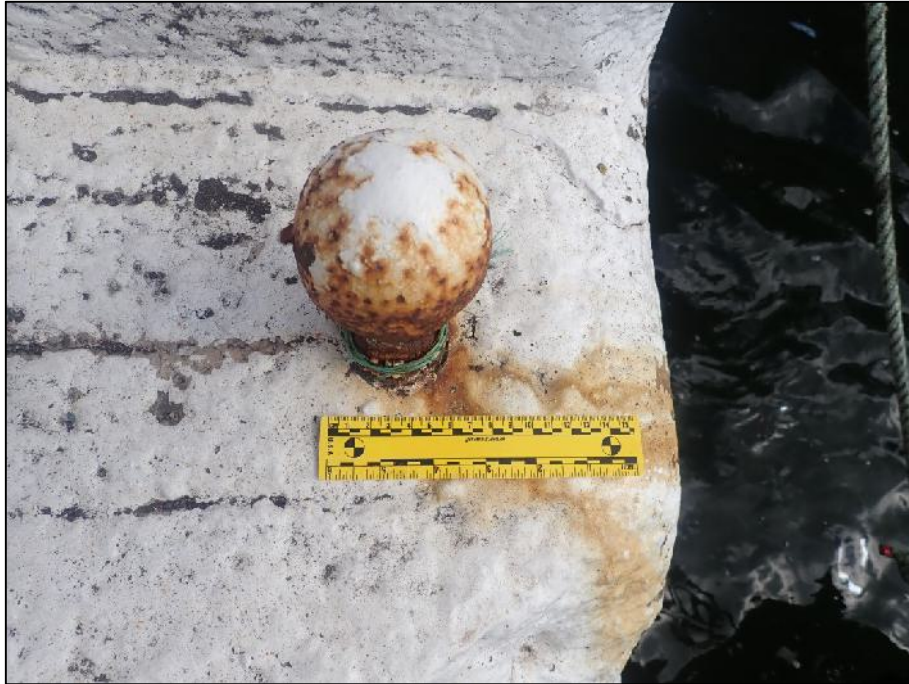
Plate 17: Detail shot showing example of boat tie-off fitting, inset into every second step (150mm scale).
