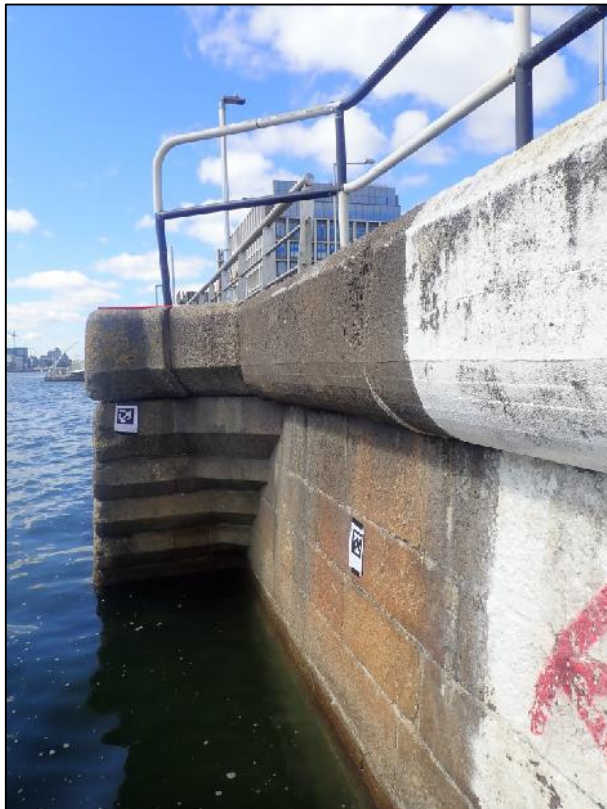
Plate 18: West-facing view of bullnose terminus to cascading masonry on the upstream side of river access steps (RAS01).
