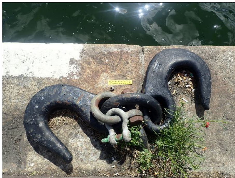
Plate 11: Mooring hook (MH03), located at ITM 717965E, 734391N (150mm scale).
