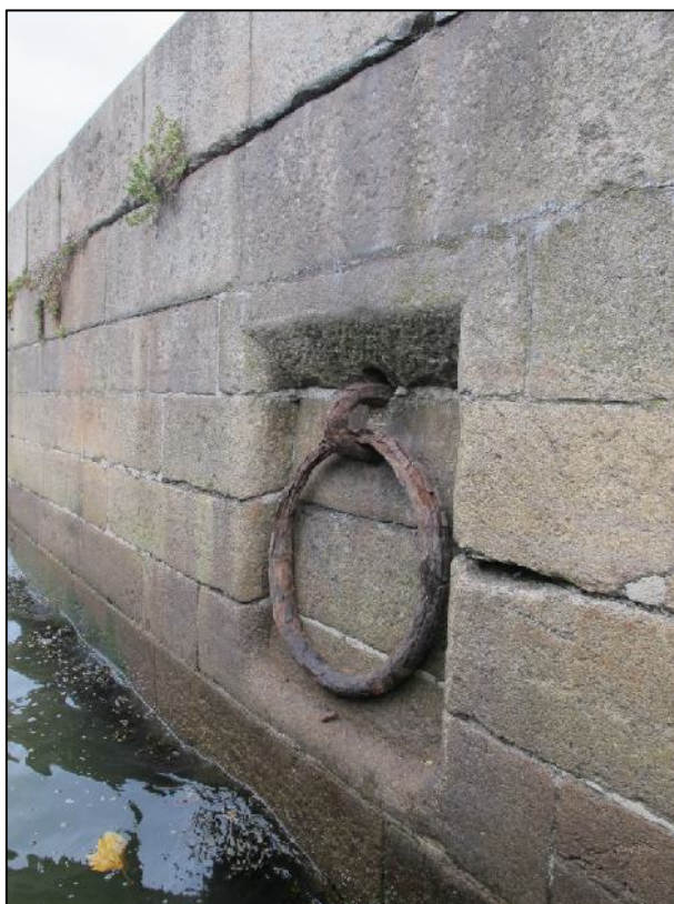
Plate 14: North-west facing view of recessed mooring ring (MR01).
