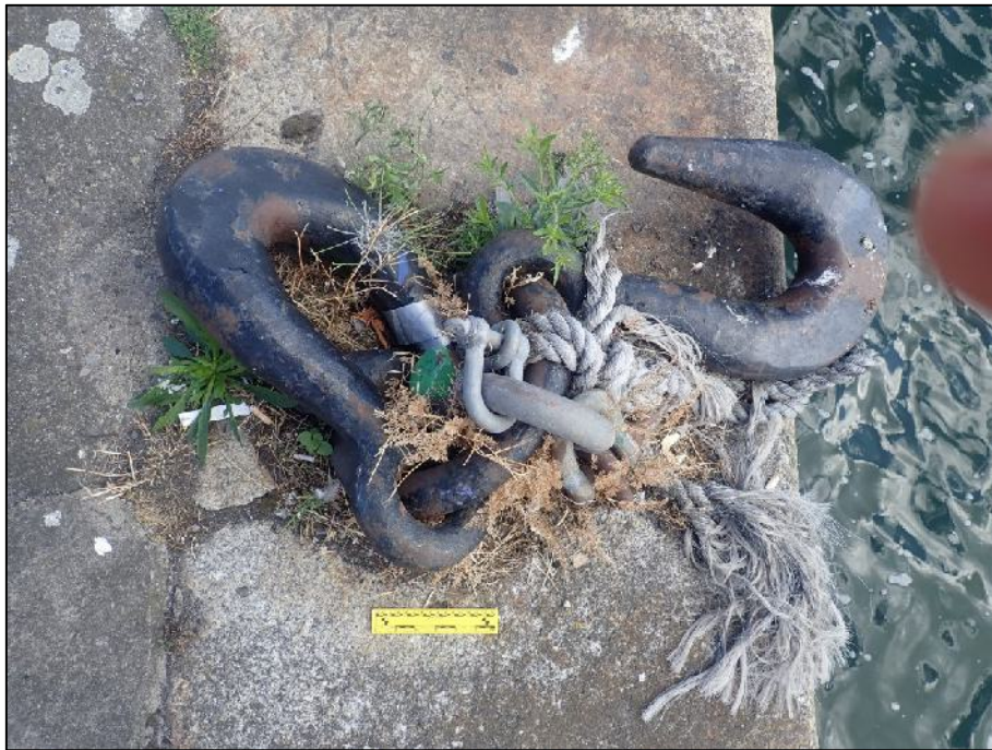
Plate 9: Mooring hook (MH01), located at ITM 718002E, 734387N (150mm scale).
