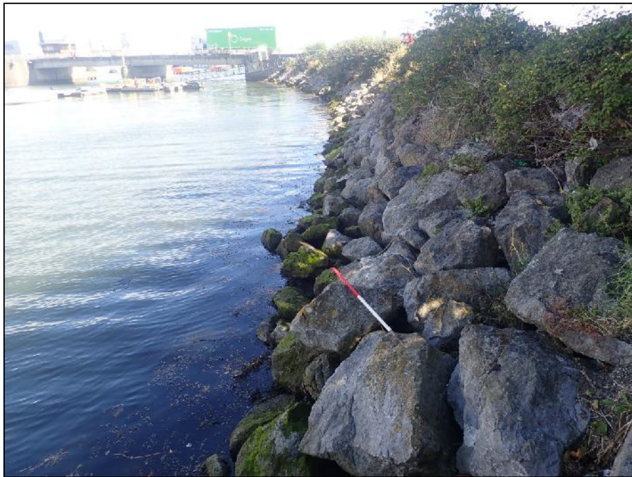
Plate 21: East-facing view along rock-armour that delineates the southern shoreline on the upstream side of Tom Clarke Bridge (1m scale).
