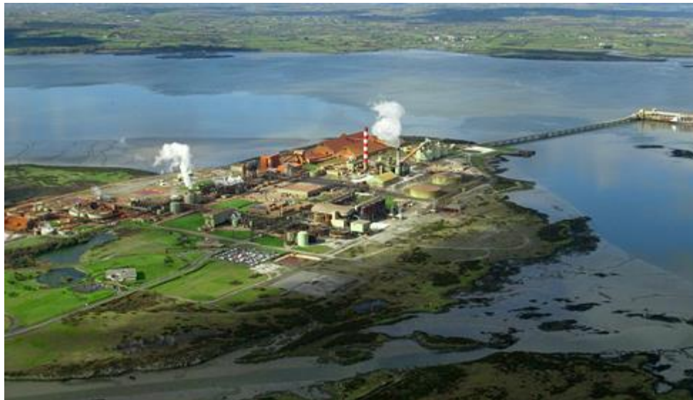
Photograph 5-1: View of refinery with deep water jetty
