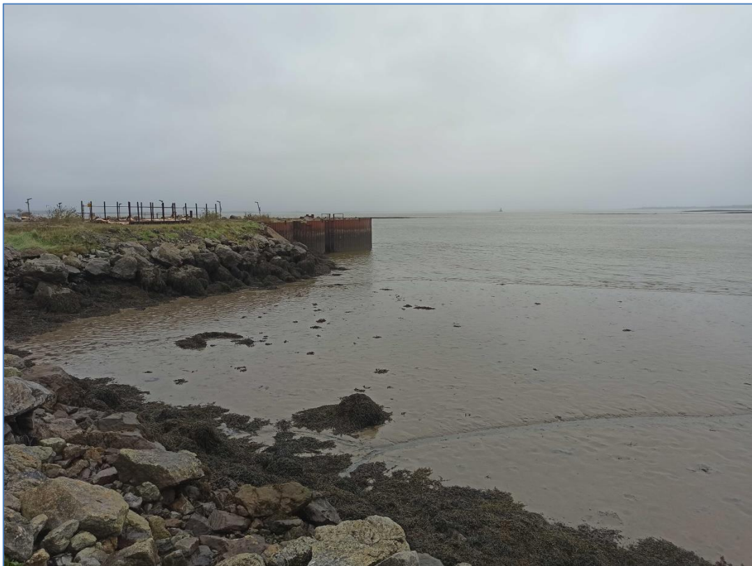
Plate 5: View from south of service area with rock armour and mud flats to the south (LDARCH 2023).
