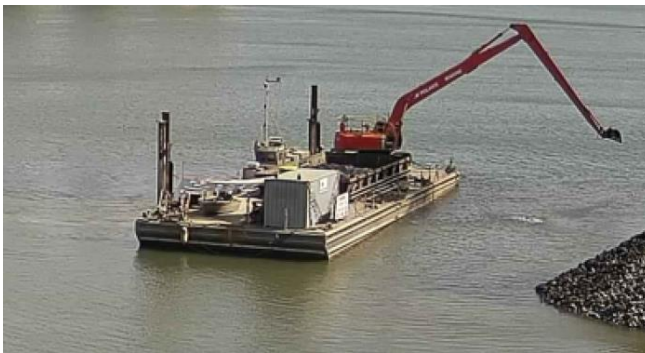
Plate 2-3: Long-Arm Reach Excavator operating from a Barge (LR/B)
