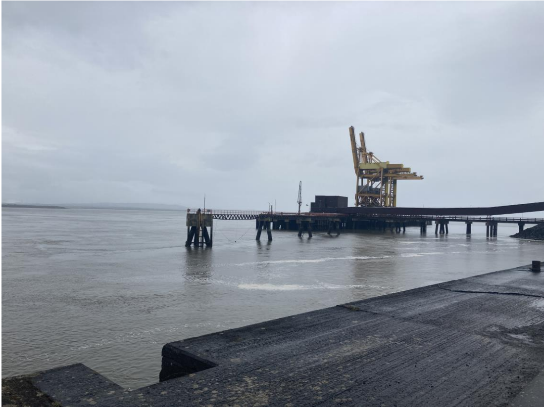
Photo 1 Existing bulk coal unloading jetty and link bridge ashore (BMcD 11/04/2024).
