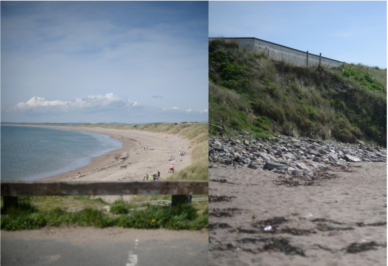
Plate 1. Beach from the car park area (L). Area beneath car park (R).
