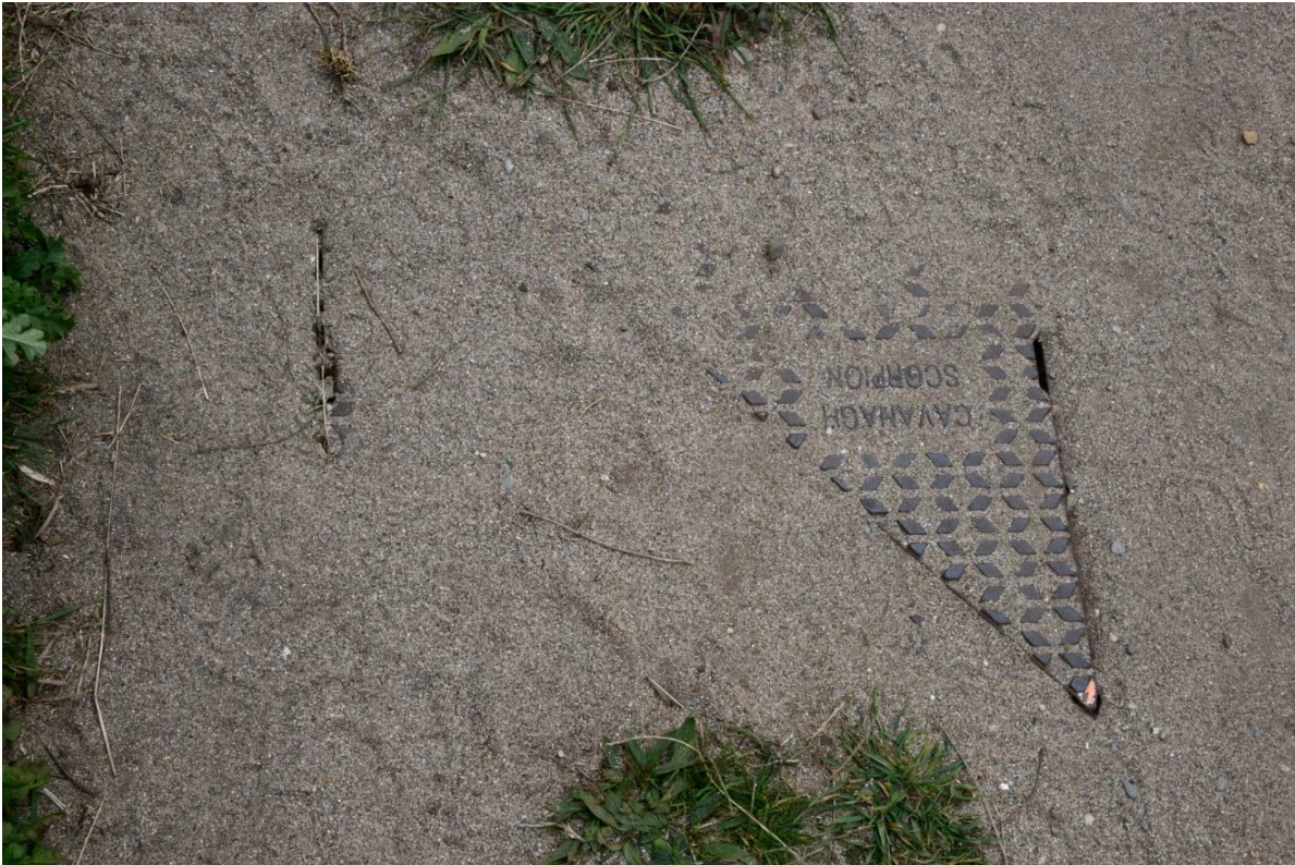
Plate 5. Existing beach manhole (not covered by dune habitat)
