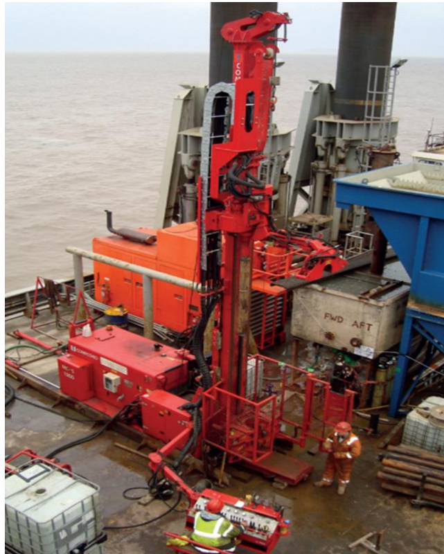
Figure 0-11: Example of a drill rig mobilised on a jack-up (Comacchio MC1200)
